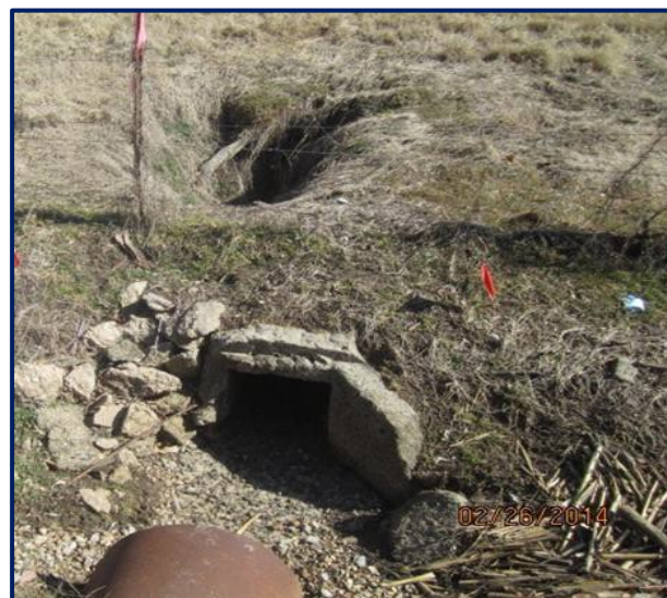
One of several culverts to be replaced along the Farrenburg Levee
